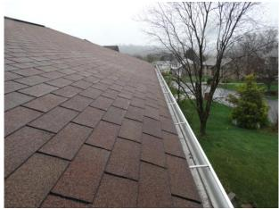
A shingle was missing from the lower left roof. The missing shingle should be replaced.
